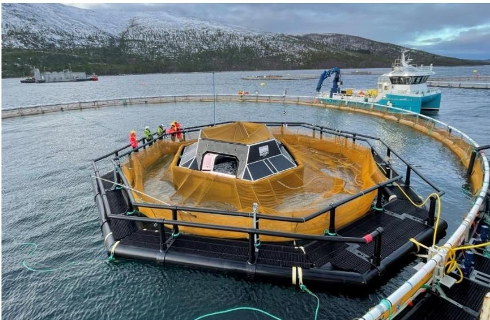
Figure 13 showing the iFarm house with one sensor unit (visible with lights) and two dummy openings being installed in cage M3.
