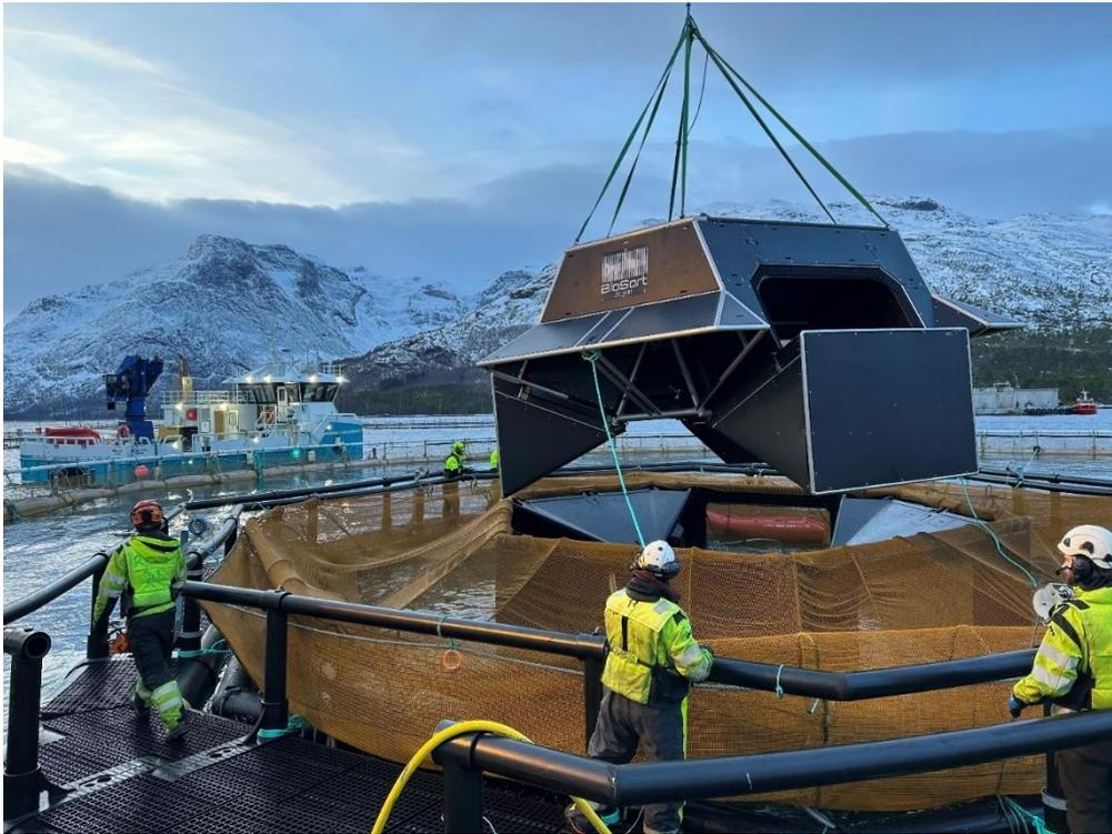
Figure 12 showing the iFarm house with one sensor unit and two dummy openings installed in Hellarvika cage M3.
