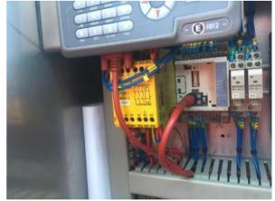
I made an assumption that the comm error was between the din mounted PLC and the HMI. So I powered off the system, removed the circular connector end of the red cable, and cleaned the contact pins. After this the system booted correctly with no comm error, and immediately showed 14.00 mm.
